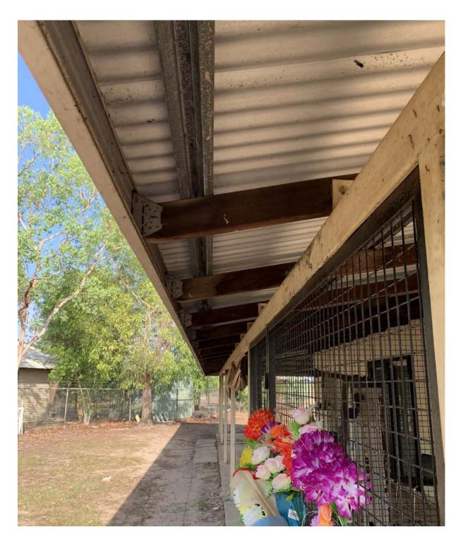
Figure 1. The veranda, posts, beam, the mesh and the 200mm gap between beam and iron roof
