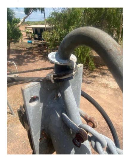
Figure 4. Showing braided cable touching plate on riser and insulated collar positioned below mounting disk
