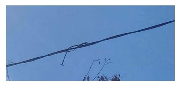
Figure 6. Showing insulation degradation on the service conductor
