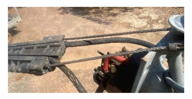
Figure 3. Showing clamp, degraded insulation and service conductors not shaped away from metal contact points
