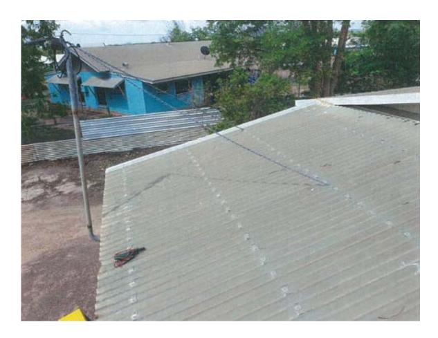
Figure 5. Showing riser and support chains connecting to iron roof
